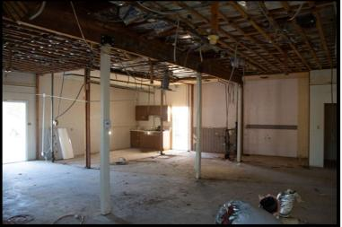
The original building preparation continues with removal of the tile ceiling and the obsolete interior walls.
