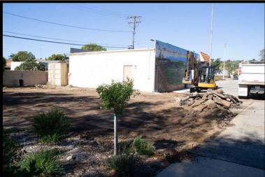
The first layer of topsoil and asphalt are cleared to begin soil compaction for the expansion building's concrete pad.
