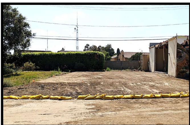
The pad for the new addition has been compacted and ready for the slab!
