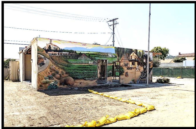
South-East corner view of the museum building. The south wall (far left) has had a section cutout to provide for a passageway into the expansion building.
