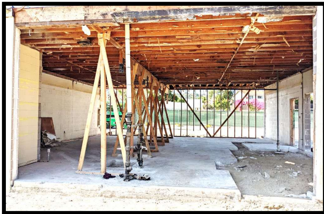
View of the south wall cutout. Temporary bracing is added inside the building to support the weight of the roof until new load bearing posts are installed.
