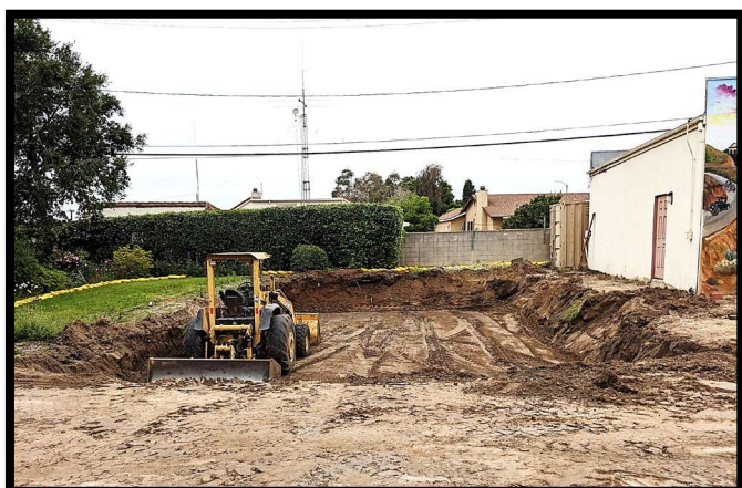
Soil below the area for the new expansion building pad was extracted to create an area for newly compacted soil. Compacted soil provides a stable/unified base for the new expansion building pad and foundation.
