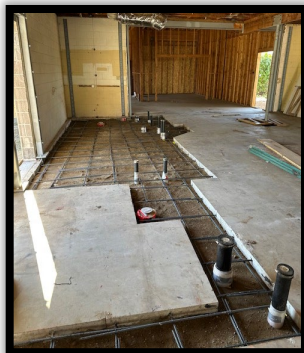
Restroom Plumbing Added
