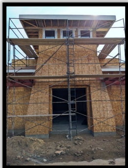
Front View of Front Tower
