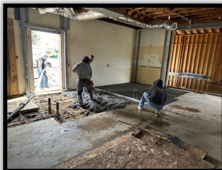
Concrete is Poured to Reestablish Floor after Restroom Plumbing is Added
