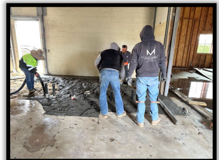
Concrete is Poured to Reestablish Floor after Restroom Plumbing is Added
