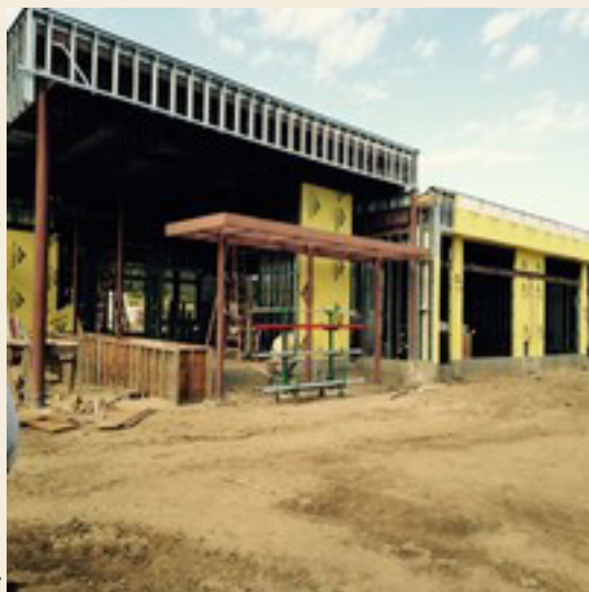
Rancho Campana under construction
